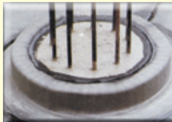
DETAIL AT PILE, USING 20% SBS MODIFIED HOMOGENOUS BITUMINOUS MEMBRANE
